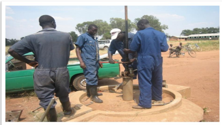
Removing the old pump
